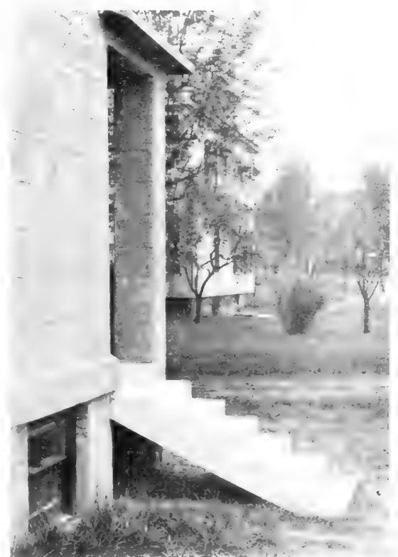
17—The Rear Outside Steps are Cast in One Form
